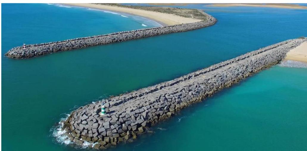
*Fig. 1 Two rubble mound breakwaters in Alvor*
