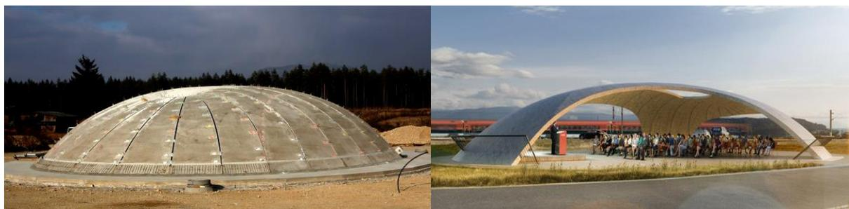
*Fig. 2 Pavilion after lifting process (left), planed end state (right)*
