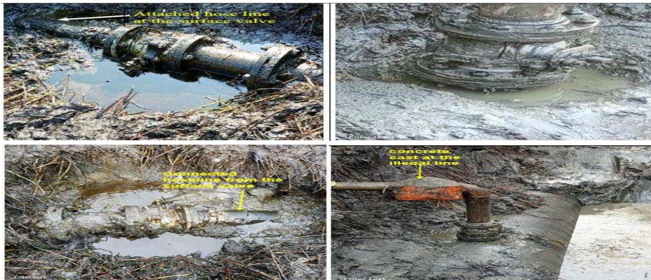
**Tapped Point and Illegal Line Connected to the Main Pipeline**
