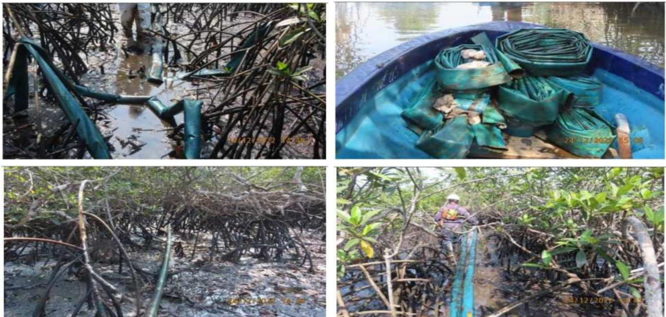
**Discovered Siphon Hoses Destroyed During Pipelines ROW Surveillance**
