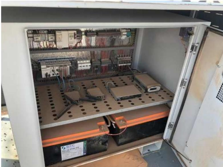
*Figure 2: : KSA-CORS IP66 Internal Cabinet filled with Dust*
