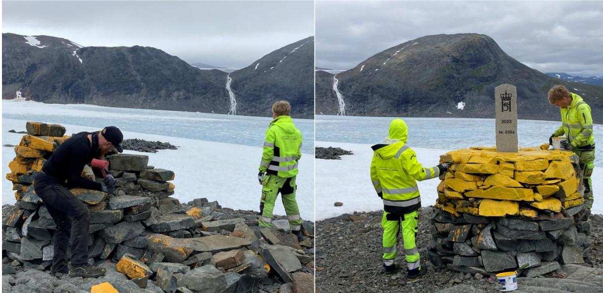
**Figure 5:** Boundary marker no 239a had by snow and hard weather been destroyed including the flat stone with the engraved royal monograms and the need for restoration was huge.
